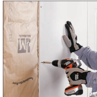
Faced fiberglass batts must always be installed with the facing correctly oriented to avoid moisture problems.
