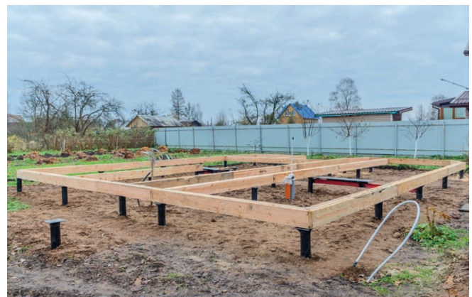
Screw piers are more tolerant of ground movement and stress than poured concrete is.
